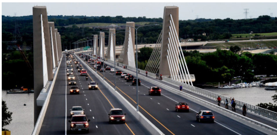
St. Croix Crossing River Crossing (STH 64)
