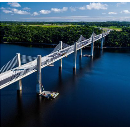
St. Croix River Crossing
