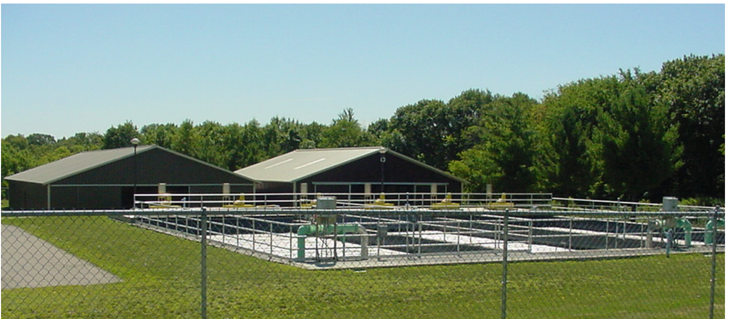
New Richmond WWTP
