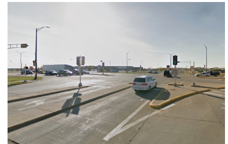
Intersection of Knowles Avenue and Richmond Way
